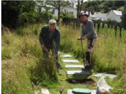
Martyn Fry and David Netherway installing the new Stepping Stone Path
